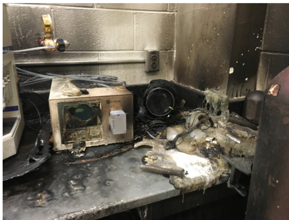
Damage to the work bench from the Lab Fire
