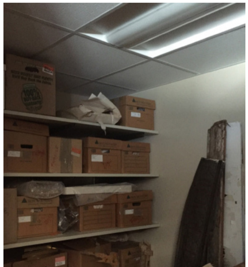
Example of boxes on shelving units reaching to the ceiling blocking the fire sprinklers
