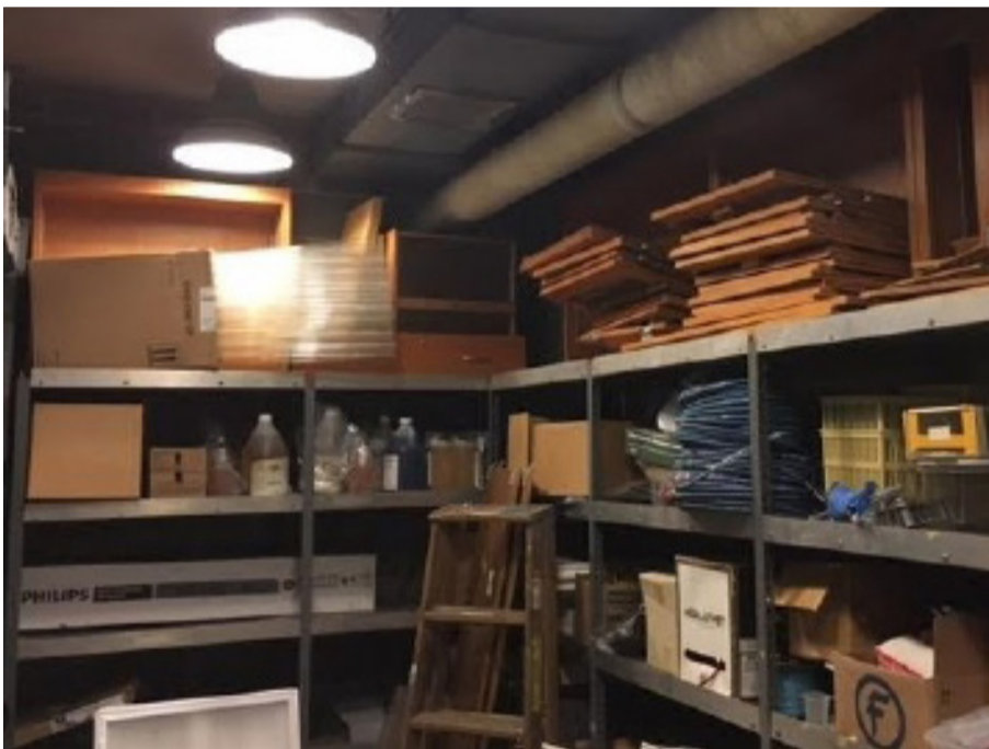
Example of closet clutter blocking fire sprinklers
