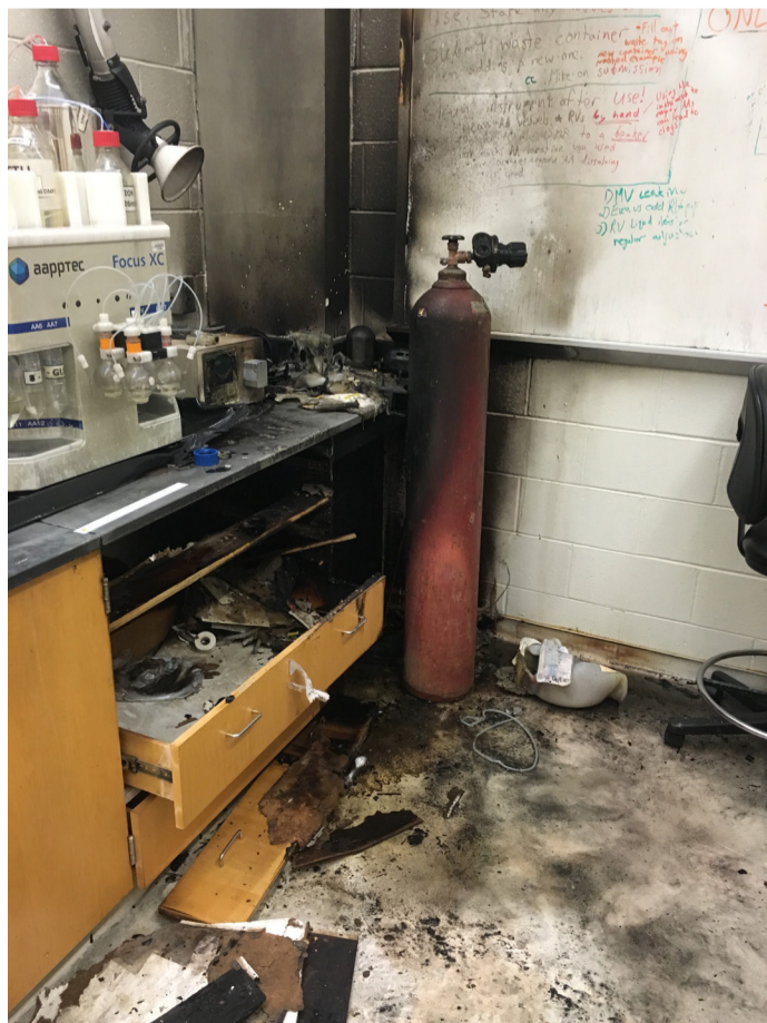
Damage from the Lab Fire
